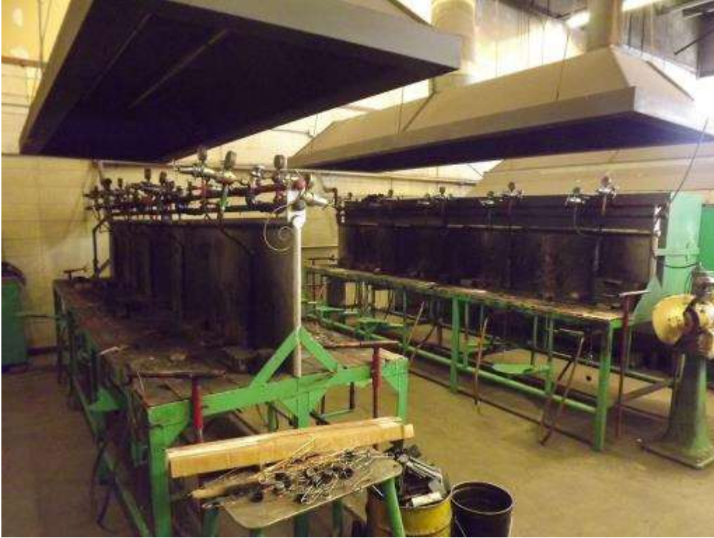
Figure 44: Gas Cutting and Welding Area
