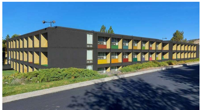
Exterior paint color options for the original residence hall
