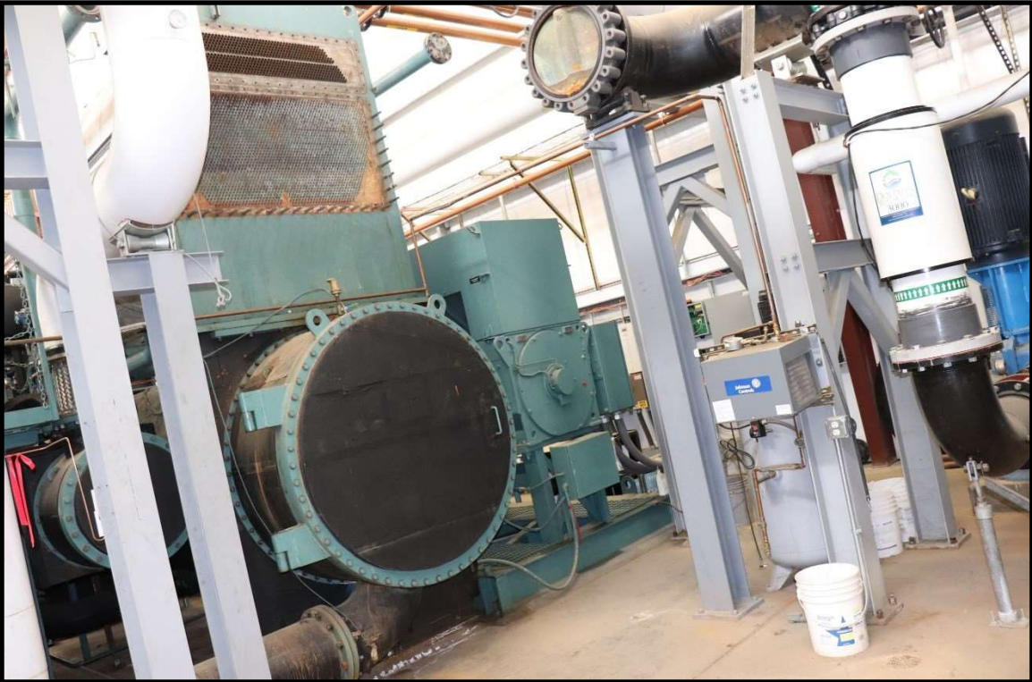
Figure 2 The opposite end as shown in Figure 1 showing partly disassembled system
