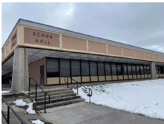
Figure 1: Upward Deflection at Eave
